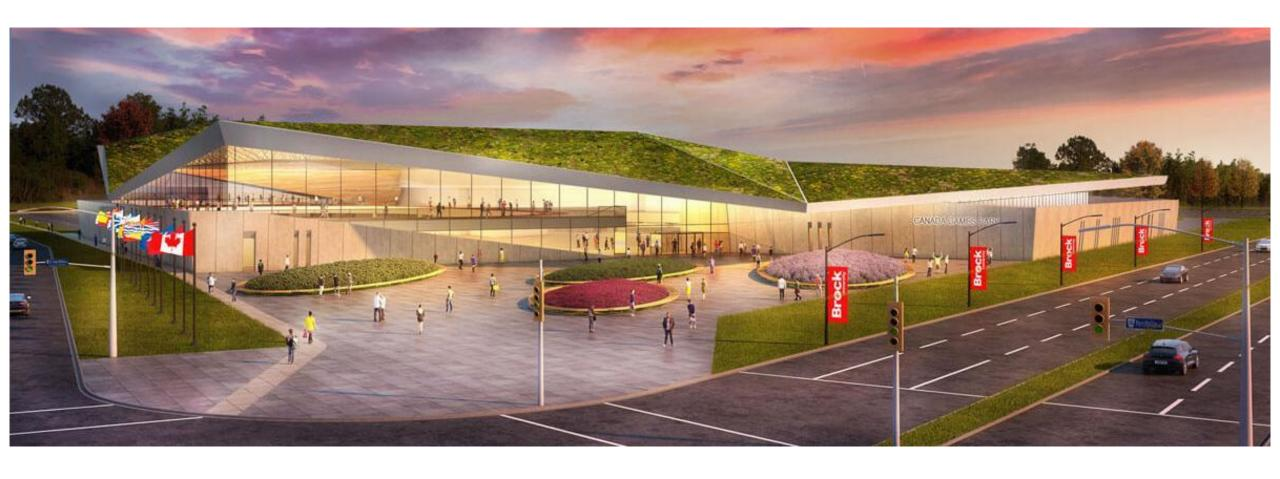
The "green roof" will help control stormwater and the urban heat island effect while reducing energy costs, and that's made possible by the way the building was designed – 35% more efficient and generating 45% less GHG emissions than standard buildings.
